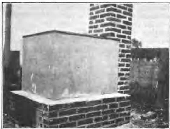
FIGURE 4.—Galvanized-iron box for heating water and for treating utensils to kill bacteria
